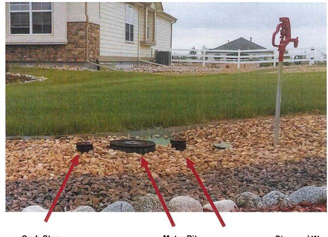
Curb Stop Meter Pit Stop and Waste Valve
